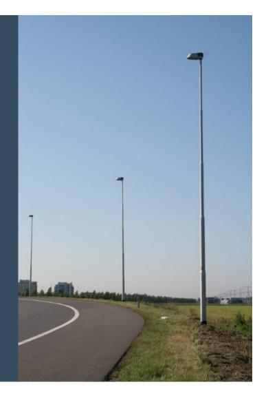
Low energy absorbing (LE) poles show the behavior that lies between high energy absorbing (HE) and non energy absorbing (NE) poles in the event of a collision.
